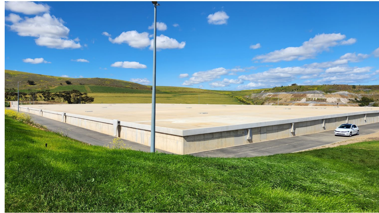
Completed Contermanskloof reservoir
